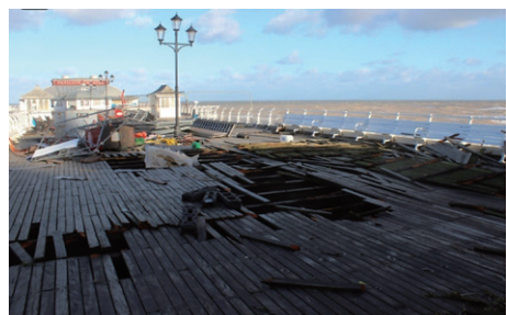
Cromer pier decking damage
